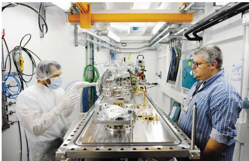
Installation of a mirror in the optics hutch of the DEIMOS beamline.
