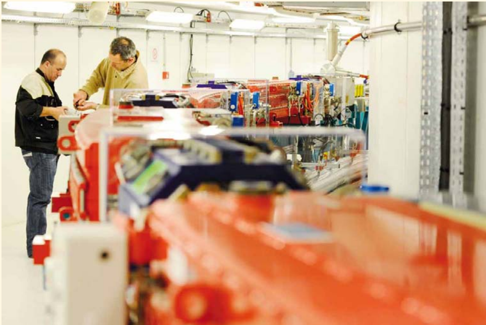
In the booster tunnel.
